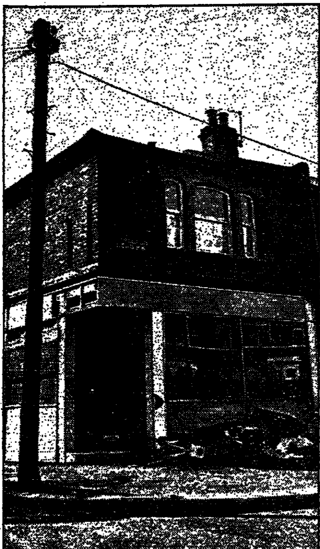
For years special finance has been available through the Society to help fight deterioration in the housing stock. Nationwide was the first Society to launch a special support lending scheme in a housing action area, Brent (above). For instance, this former shop will be converted to living accommodation. To help further, the Society has sponsored the Nationwide Housing Trust Ltd which is undertaking direct housing development activity.
